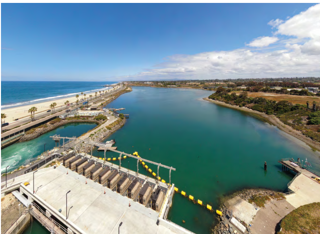
LOCAL SOLUTION The Claude "Bud" Lewis Carlsbad Desalination Plant provides a drought-resilient local supply capable of meeting approximately 10 percent of regional water demands.
